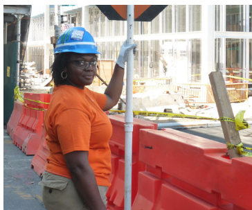
Stacy Knutt, the eighth member of her family to join Local 79 and a construction worker at Manhattanville since 2012
